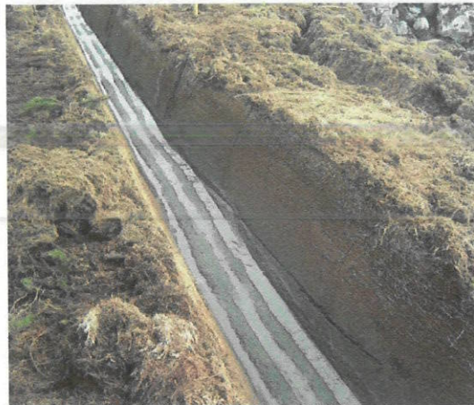
Plate 11.6 Typical drain installed during wind farm construction
